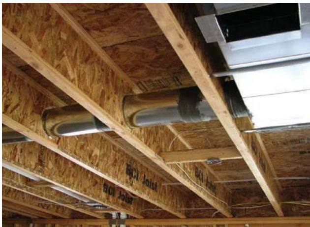
With this system, ducts and other mechanicals are protected during construction, and leave a clean finish at the end of the project.
